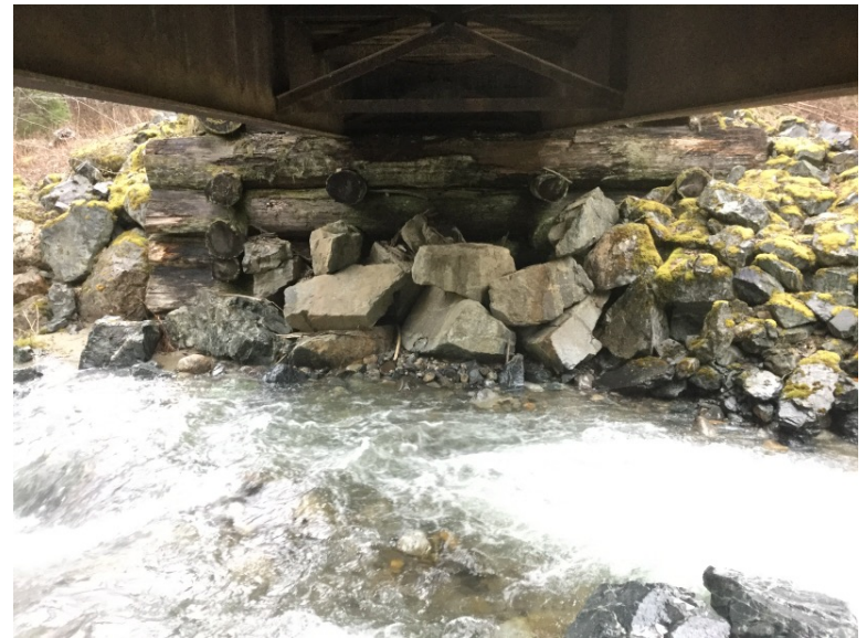
Right Bank Abutment when facing downstream
