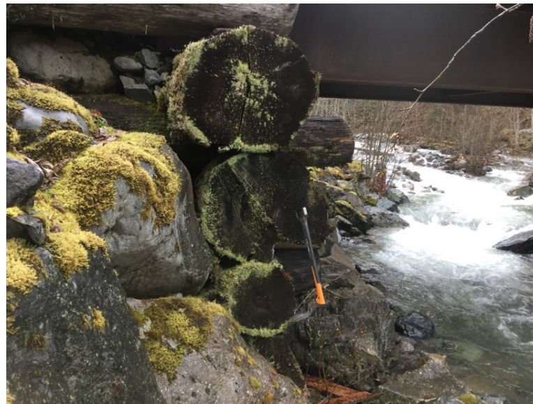
Downstream right bank face log ends
