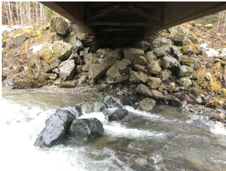
Left Bank Abutment when facing downstream
